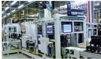
Manufactory Monitor System
